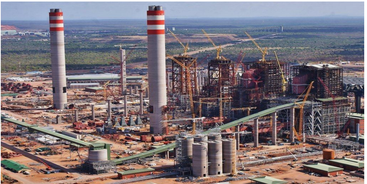
Figure 1: Construction at Medupi Power Station
